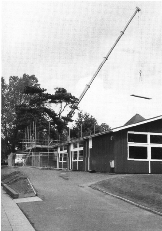
The New Geography and Business Studies Building Top: Architect's drawing of the south front of the building Above left: The suspended floor is laid Above: The roof level takes shape Left: A crane lifts the floor blocks into place Right and below: Two views of the completed building
