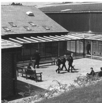
New Changing Room complex and OBS piazza.
