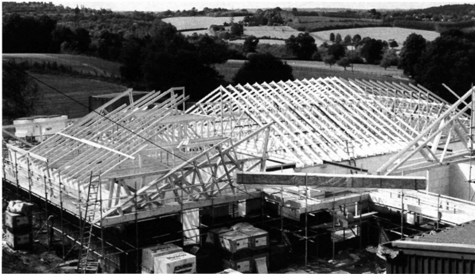
Below: The roof trusses are lowered into place.
