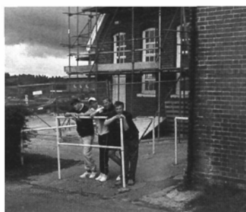
Scaffolding around South Wing – building renovation.
